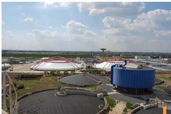
Valenton (94) Station d'épuration
