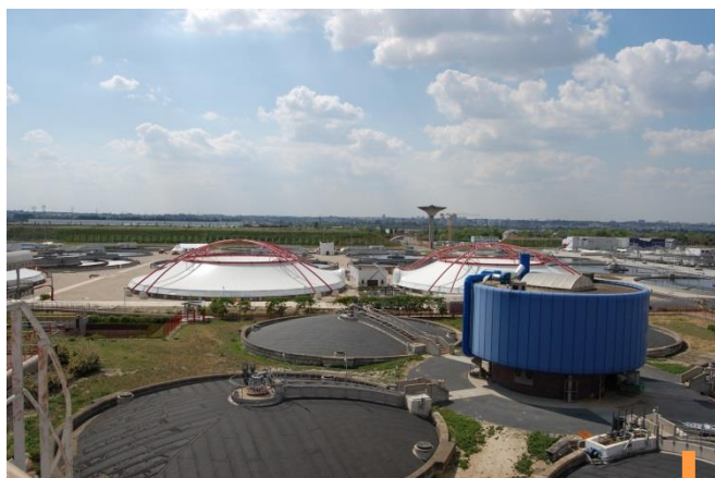
Valenton (94) Station d'épuration
