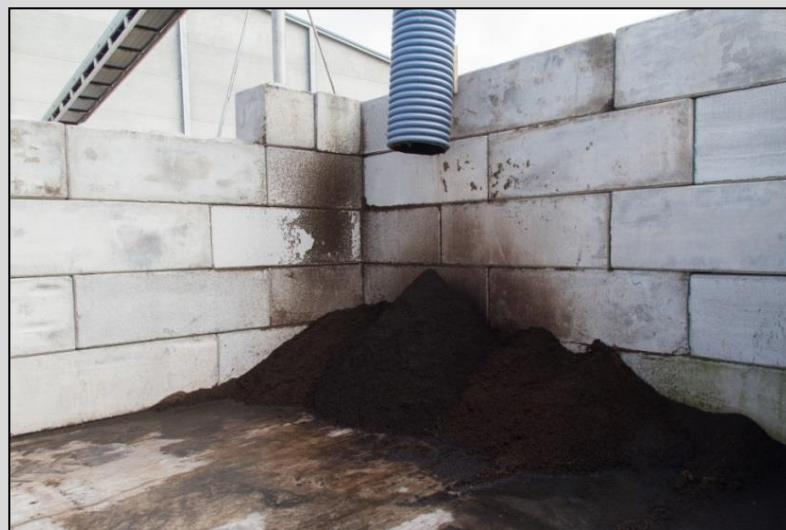
Stockage digestat solide
