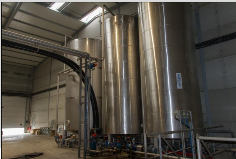
Stockage extraction digestats
